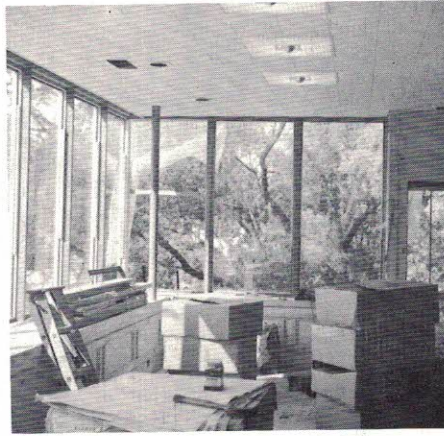
Mr. Herbert W. Armstrong's new office nears completion.
